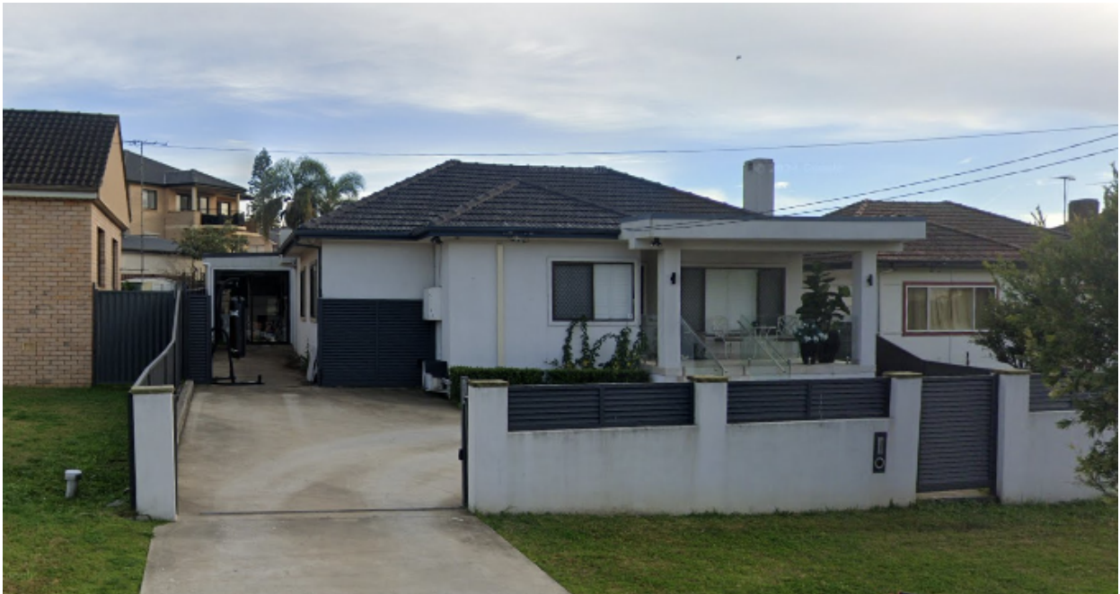
Figure 2: Street View of No.50 Rea Street, Greenacre
